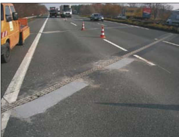
A2 Motorway, Bielefeld: Repair of transverse drainage channels
