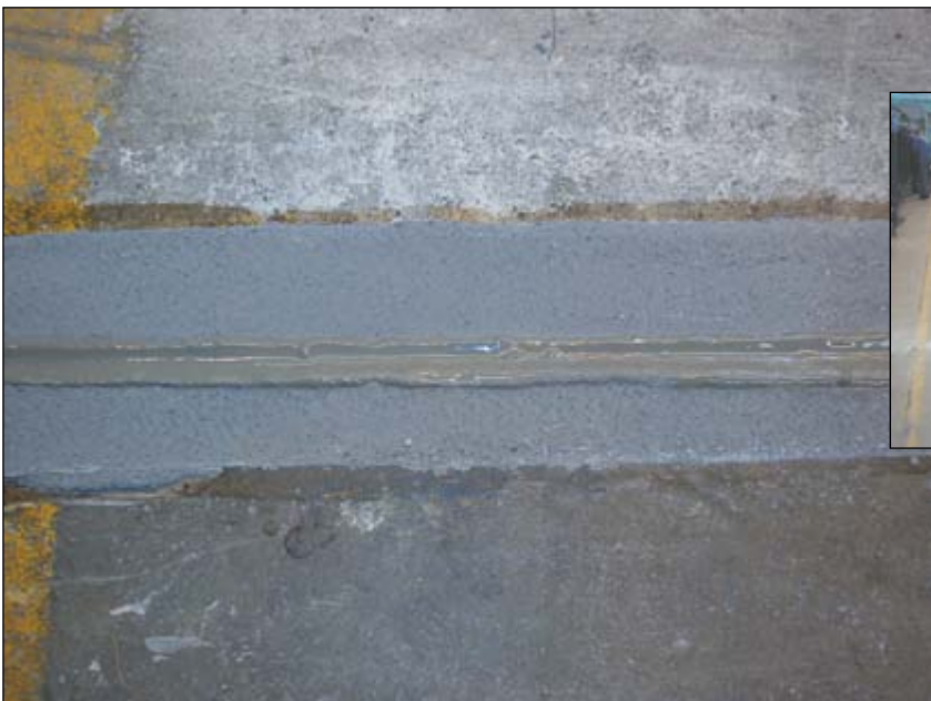
Left: Rheingas AG, Brühl: Repairing sliding gate
