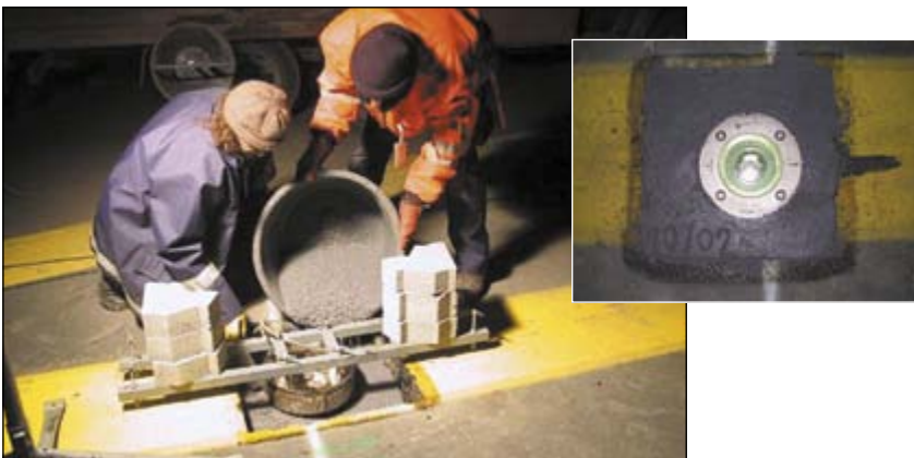
Nordrhein-Westfalen Airport: Replacing and installing embedded runway lights without air-traffic interruption
