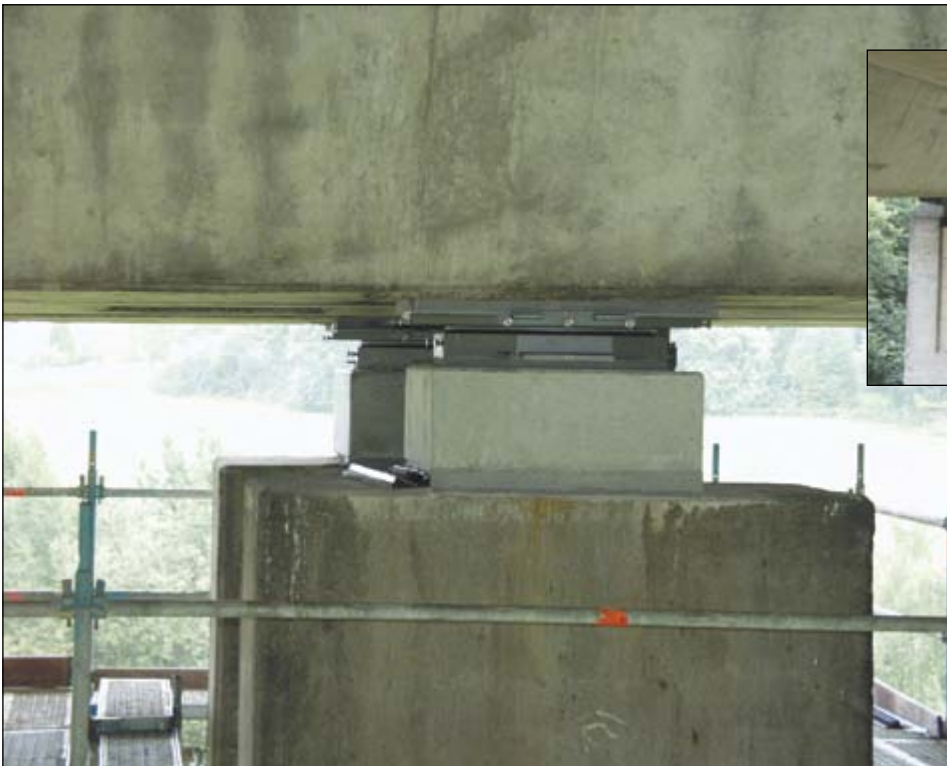
A7 motorway bridge, Uttrichshausen: Repairing bridge bearings
