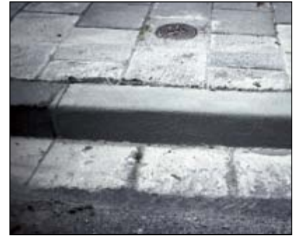
Repairing the kerbs with SILIKAL® Mortar R 17
