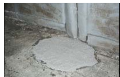
Figure on top: Deutsche See GmbH & Co. KG, Bremerhaven: Repair of floor areas in cold store house with SILIKAL® R 17 mortar with no disruption to operation (-25 °C)
