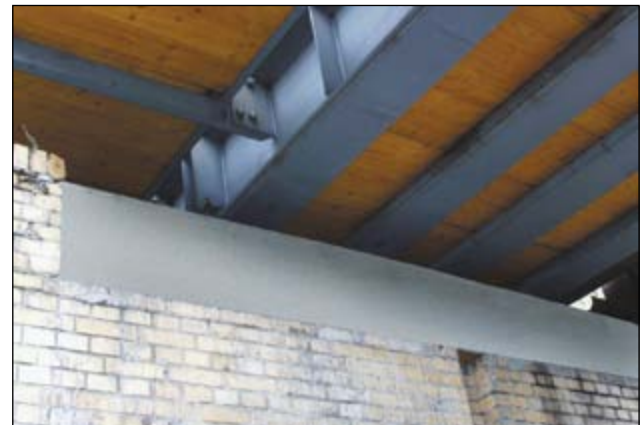
Metropolitan viaduct, Berlin, Sterndamm: repairing bridge bearings
