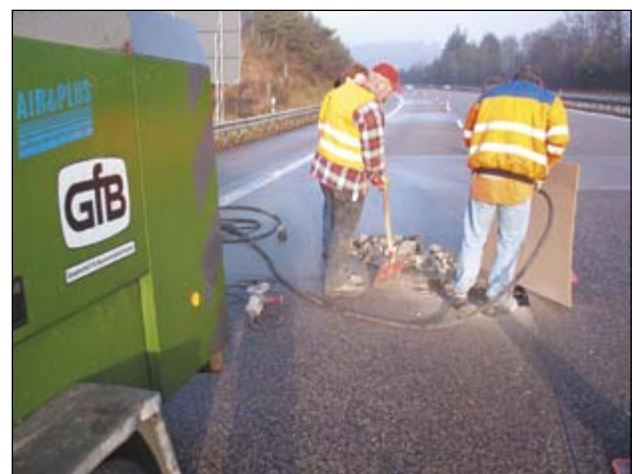
A3 Motorway, Neustadt/Wied: Improving the road surface
